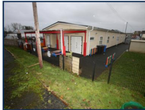
Lack of external play space
