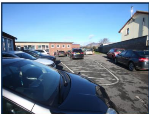
Access problems at entrance and lack of parking facilities for staff & parents
