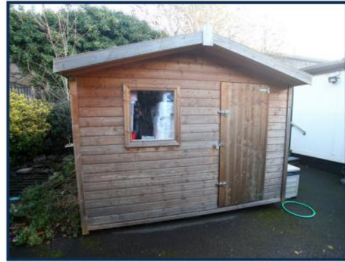
Timber shed as school store
