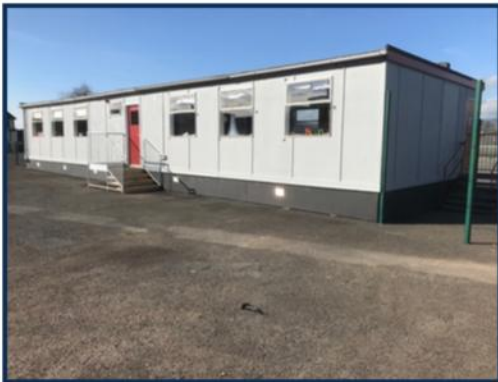
External areas - level access not provided to all classroom units
