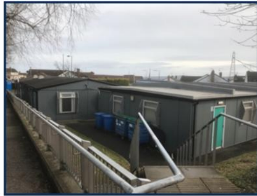
Access via steps
