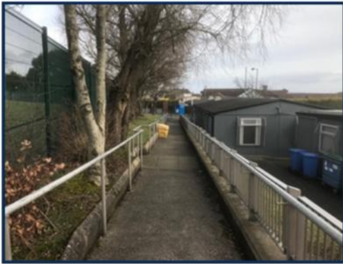
Ramp access to school admin building
