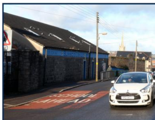
View from main road to the emergency exit
