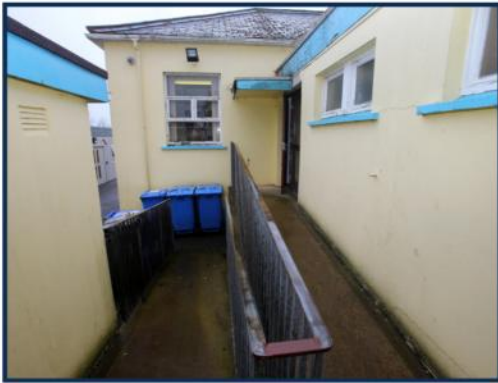
Access point to classrooms
