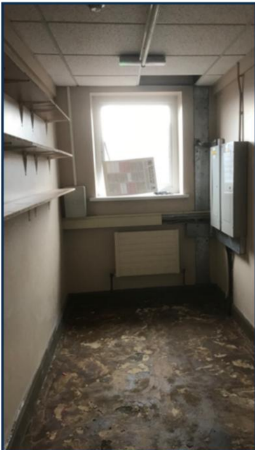
Store to be converted to sensory room
