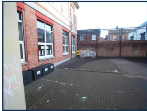
Hard play area at rear of building
