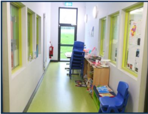
Lack of storage for classroom equipment
